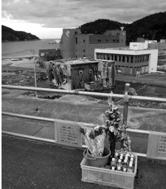
In Onagawa, just a 10-minute drive from Watanoha, the tsunami reached 17.42 m, inundating the first floor of the hospital. People standing beside this little shrine all perished. Concrete buildings like the one shown below it were ripped from their foundations and hurled onto their sides several meters from where they once stood.
