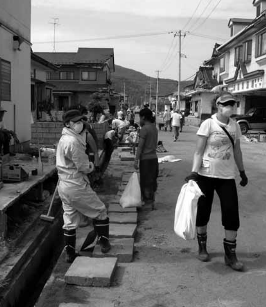
Our early trips were all spent cleaning debris out of the drainage gutters alongside the roads.
